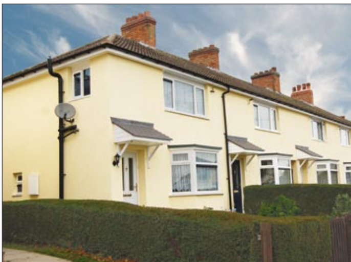
Social Housing Refurbishment Project: Heavy Duty NSC5 EWI System
